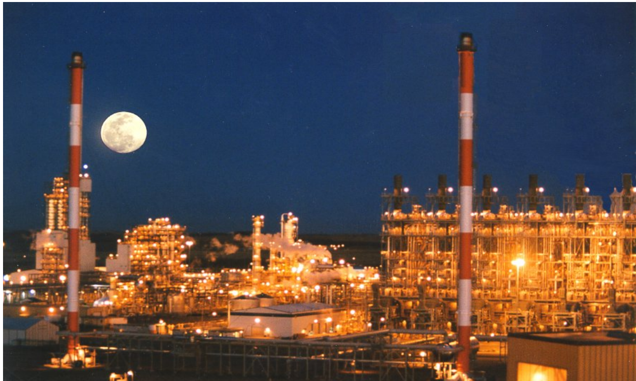
Figure 1: An Overhead View of NOVA's Advanced SCLAIRTECH polyethylene plant (PE2). Joffre, Alberta
